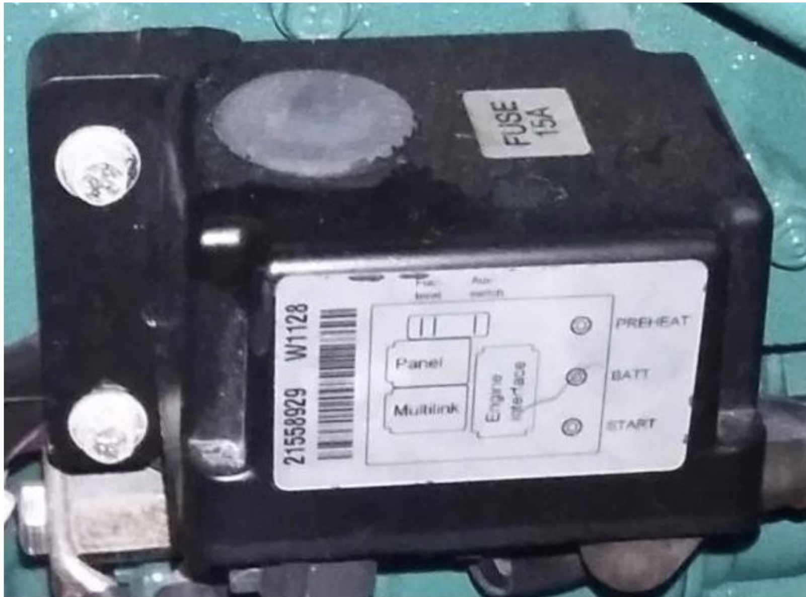
By 2011 already, a 15A blade fuse was added to the MDI box, protected by a sealed rubber cover.
